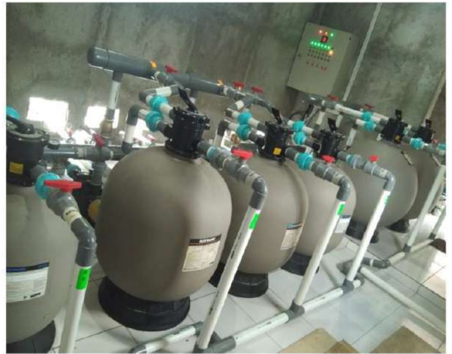
Instalasi Mesin Hayward Oase Waterpark, Kawarang Timur-JawaBarat.
