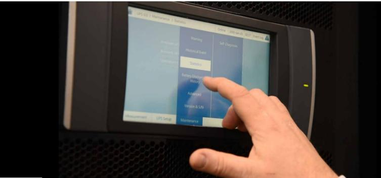
Delta's DPH series Modulon UPS offers the ability to view up to 10,000 event logs on the touch panel. The unit's 10" LCD screen can optionally display information on security, cooling, fire protection, and temperature in addition to battery status. The availability of all this information on the touchscreen of the UPS allows for easy local management.
