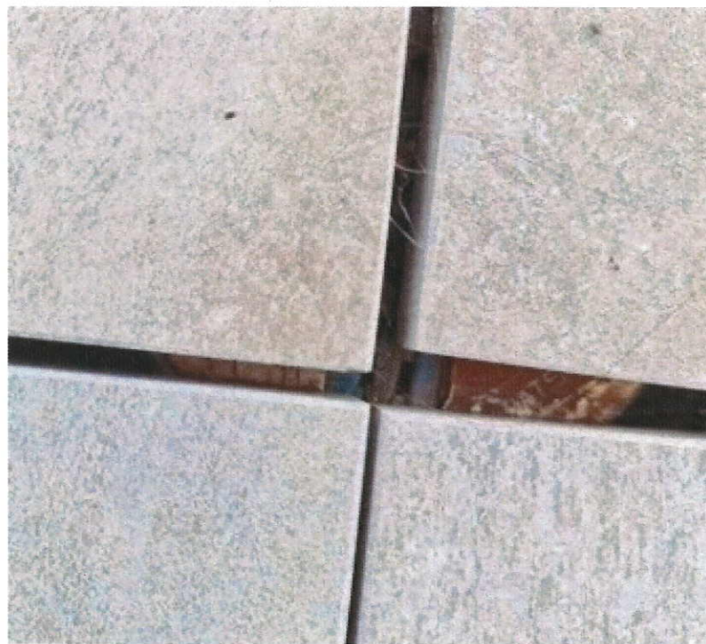
PHOTOGRAPH 10 shows missing spacer lugs
