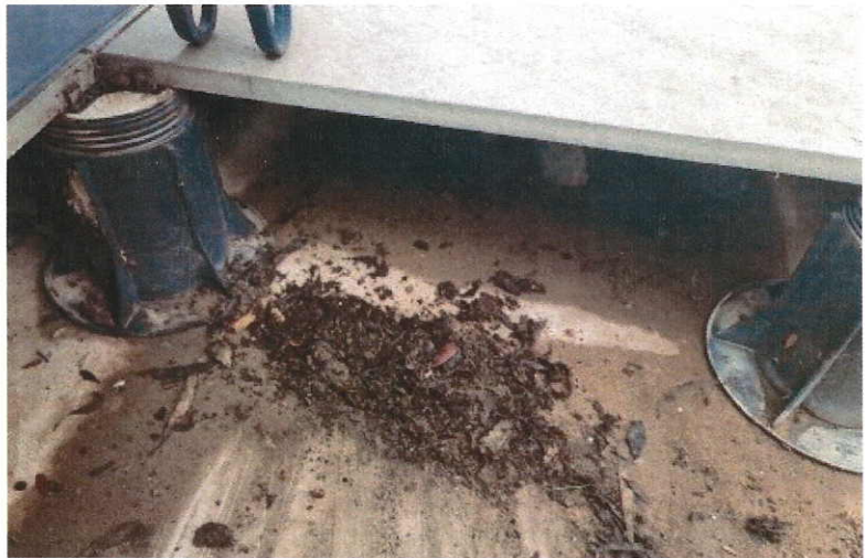
PHOTOGRAPH 4 depicts debris under a podium system two years after installation
