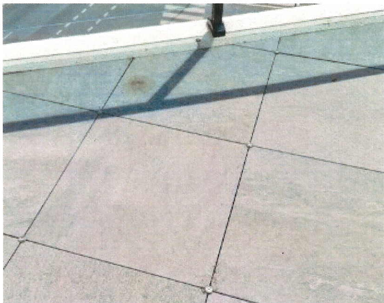
PHOTOGRAPH 2 depicts a mechanical fixing system to prevent dislodgement of tiles that were previously flipping over in high winds
