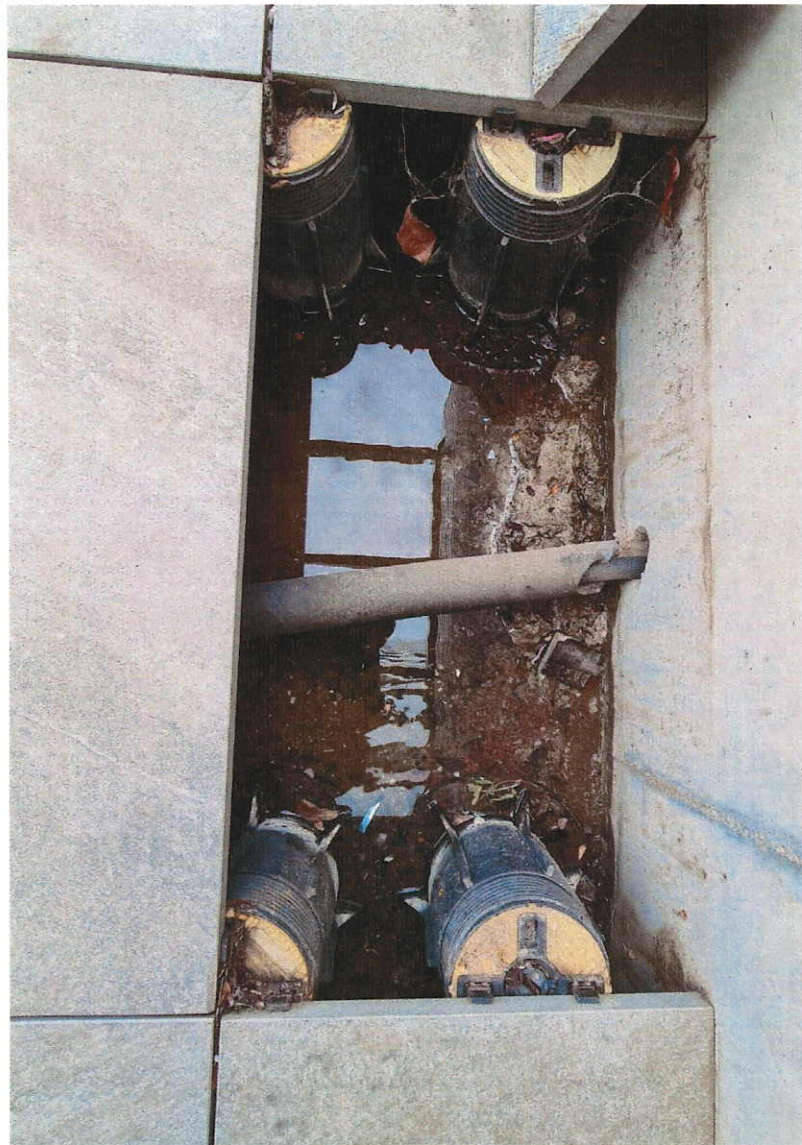
PHOTOGRAPH 11 shows water retention beneath the tiles due to insufficient gradients
