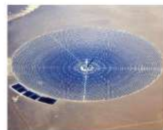
Figure 14.5 Mirrors reflect sunlight to a point in the tower (in the middle of the mirrors).
