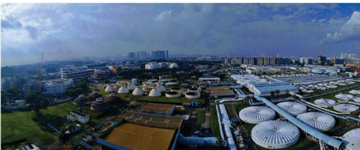
Figure 13.12 NEWater is produced from treated used water that is disinfected using UV and other processes in the water reclamation plants in Singapore.
