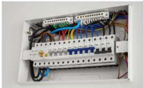
Figure 18.13 Circuit breakers of a distribution board box
