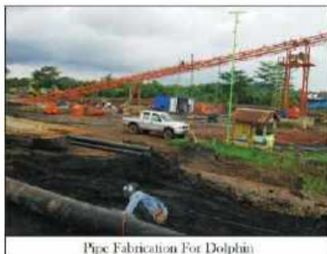
Pipe Fabrication For Dolphin
