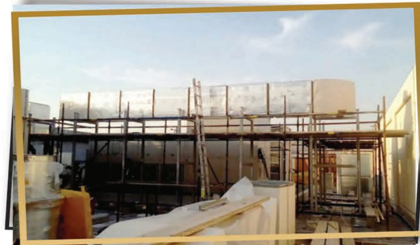
Square Duct With Bode Insulation
