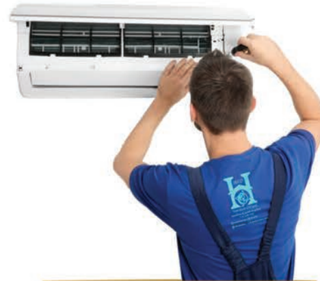
Air conditioning devices
