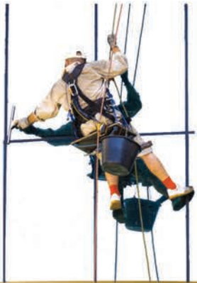
Cleaning glass facades
