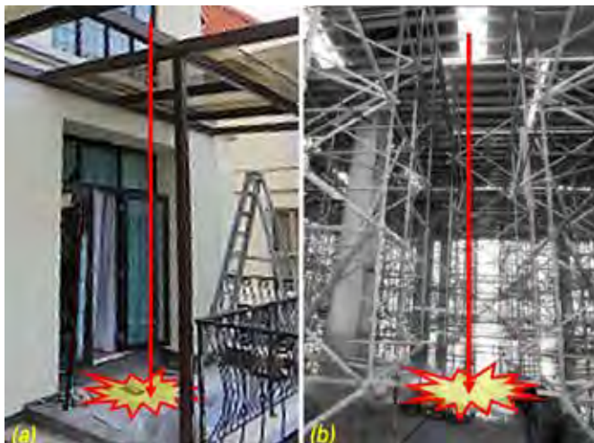
Fig. 1. (a) Fatal fall from canopy, (b) Fatal fall through formwork gap
