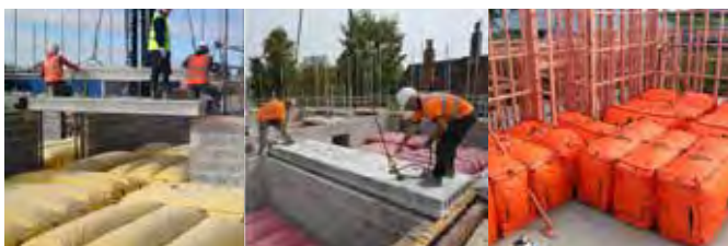
Fig. 6. Air-bags in general, concrete, and timber construction
