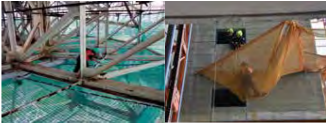
Fig. 5. (Left) Net in Steel Erection; (Right) Fallen worker caught in net.
