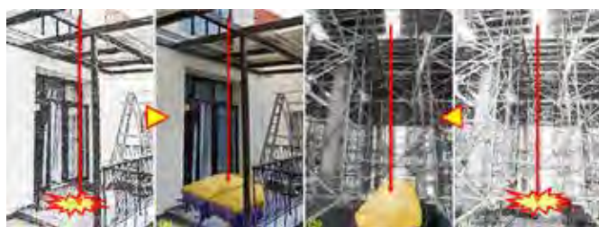
Fig. 10. Fall without and with air-bags from (a) canopy and (b) through formwork gap. (Outside figures, without air-bags, purposely blurred.)
