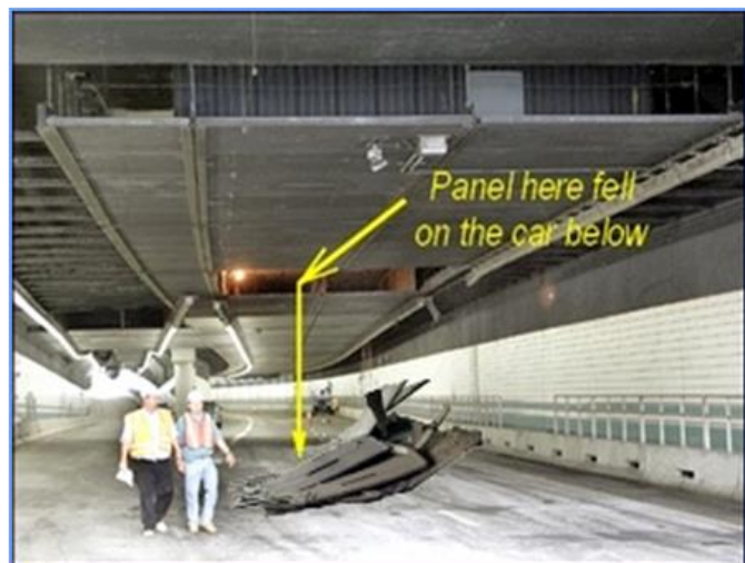
Fig. 6. Boston Tunnel Ceiling Collapse
