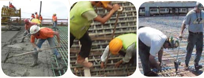
Figure 8: Left - 'bull-floating' with an awkward posture. Centre - squatting and wire binding rebars. Right - bending down and wire binding versus standing up and wire binding, using a mechanical aid.
