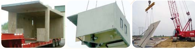
Figure 13. Left - transportation of unit. Centre - lifting of unit. Right - lifting of tilt-up slab.
