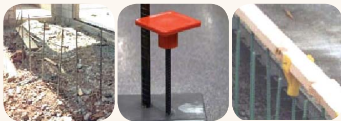
Figure 10: Left - rebar impalement hazard. Centre – plastic cap. Right - plank shield.
