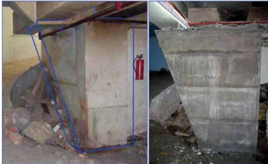
Figure 18: Column C9, (Left) Before Retrofit, with Retrofit Jacket Outline Superposed, and (Right) After Jacketing
