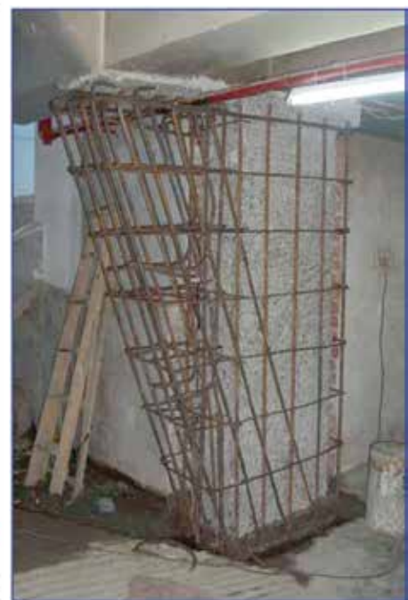
Figure 17: Jacket Reinforcement for C9
