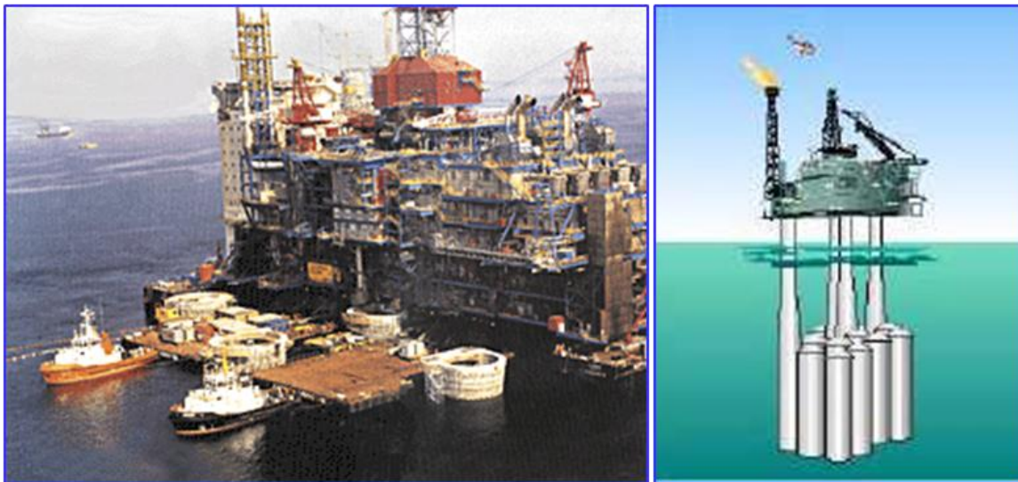
Fig. 9. Sleipner Off-shore Platform, before collapse, and schematic.
