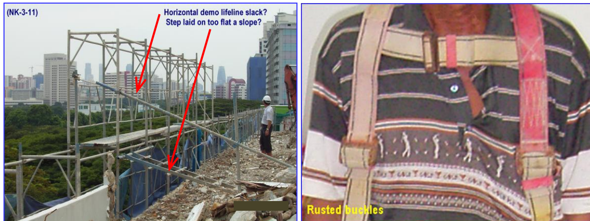
Fig.23. Specimen photos from author's investigation of worker fall
