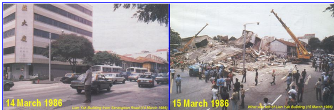
Fig. 5. Hotel New World, before and after collapse
