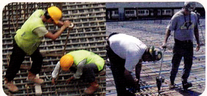
Figure 4: Binding re-bars with wire. The image on left shows a worker binding bars while in a squatting position while the image on right shows a worker standing and performing the task with the help of a mechanical aid.
