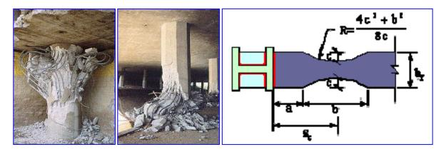
Fig. 4 (Left pair) 'Bird-caging' of top and bottom of R.C. columns; (Right) Reduced beam section in steel 'I' beams.
