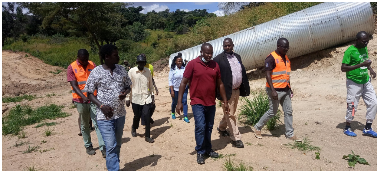
WSF, UNDP, District and Sub-county teams during the monitoring of the Loitanit-Kanadap-Nalapatui access road, in Tumu Sub County, Kaabong District.
