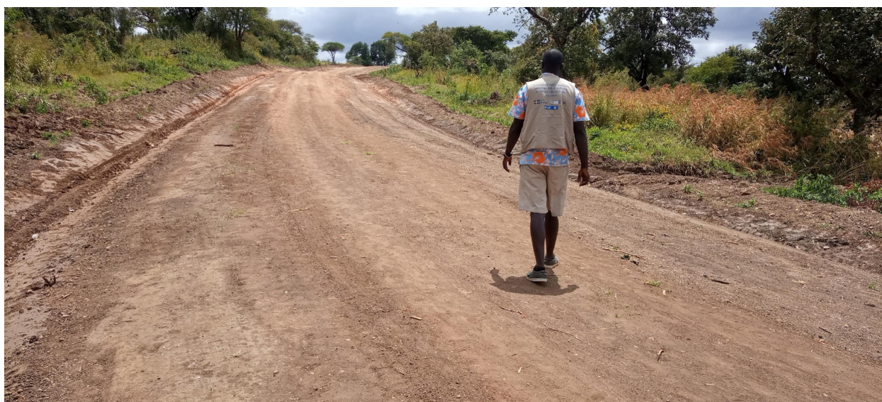
Project Engineer walking through a completed section of the Loitanit- Kanadap- Nalapatui security access road at the escarpment – 25 th Oct 2022 during the monitoring visit.
