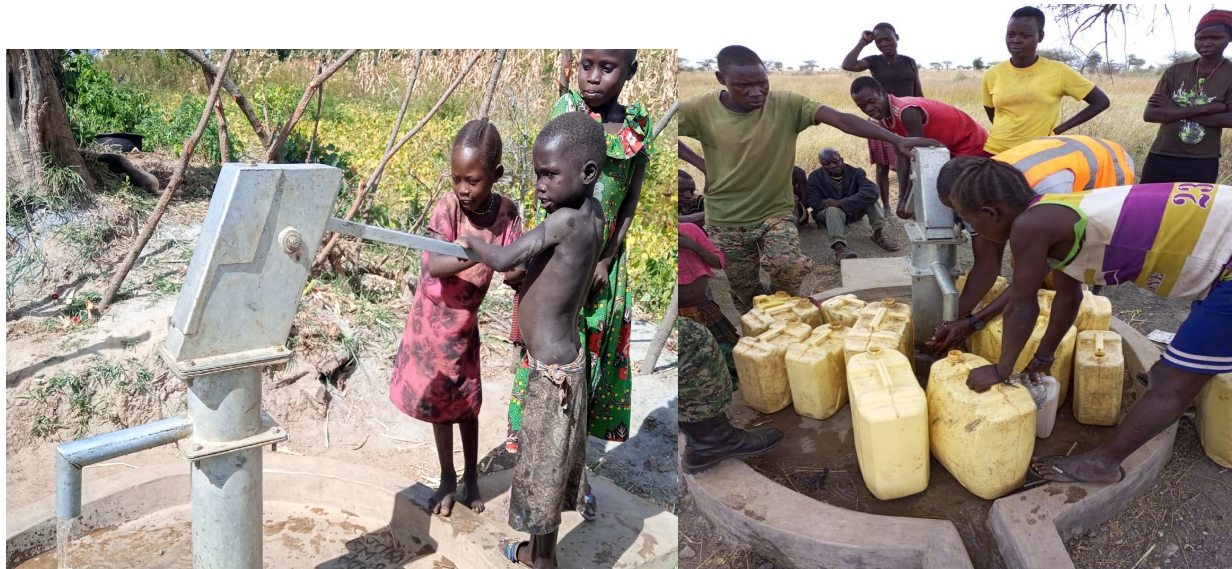
Finished installed and functional boreholes in Tultul, and Kaileny in Timu and Nakapelimoru sub-counties of Kaabong and Kotido Districts.
