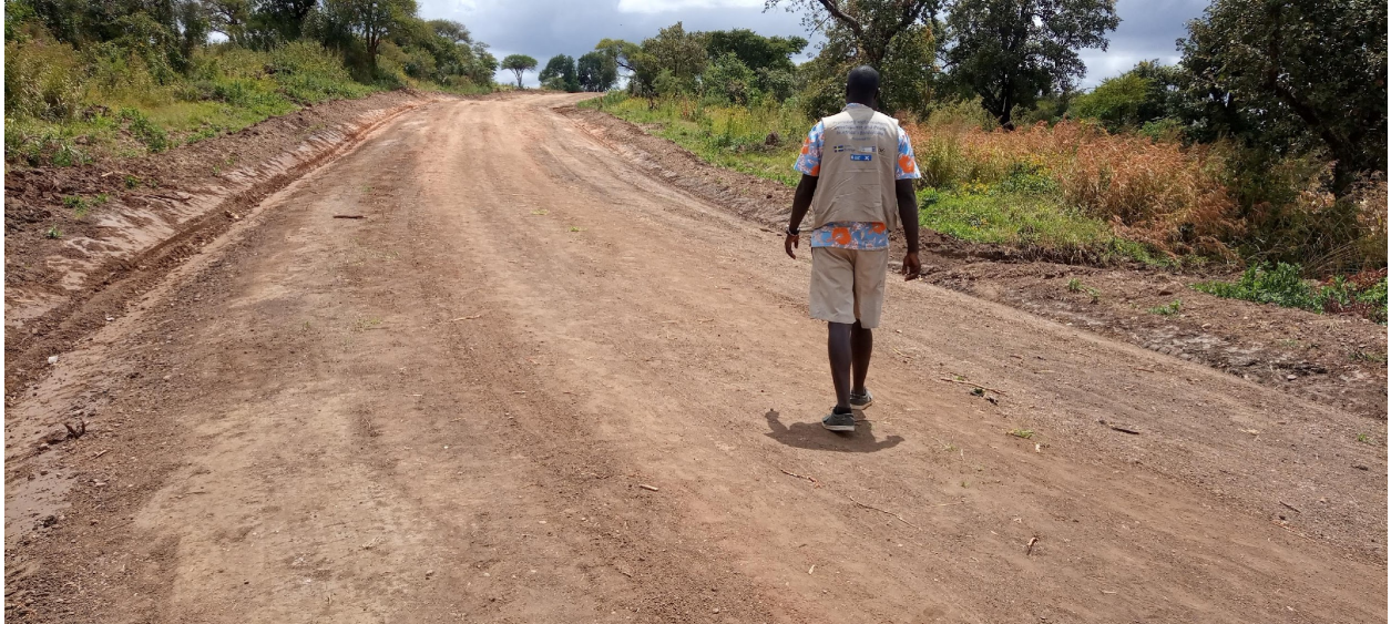
Complete cleared and graded Loitanit -Kanadap – Nalapatui road section.
