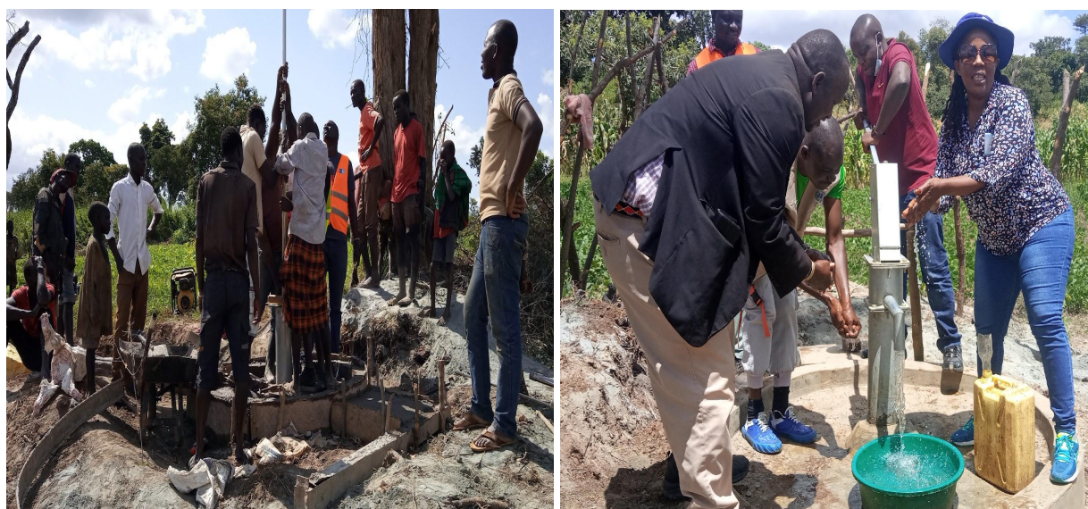
Borehole installation in Tultul, Timu Sub- County, Kaabong District and LCV – Kaabong representative, UNDP team and WSF ED during project monitoring.
