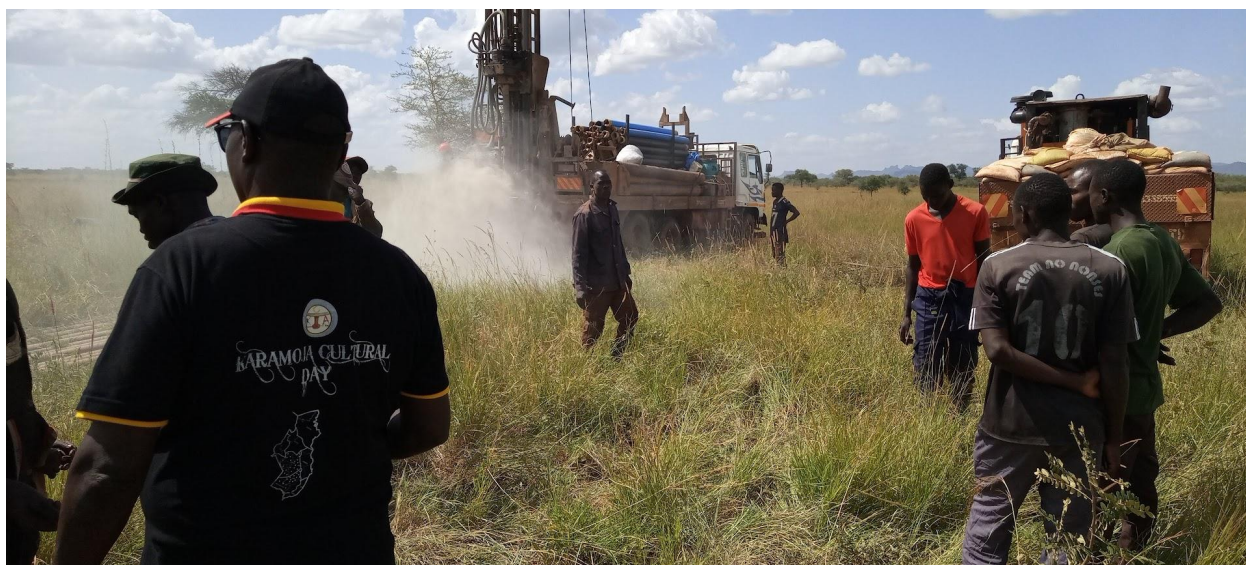
Some of the community members looking at the drilling of borehole in Kaileny, Nakapelimoru sub-county, Kotido District
