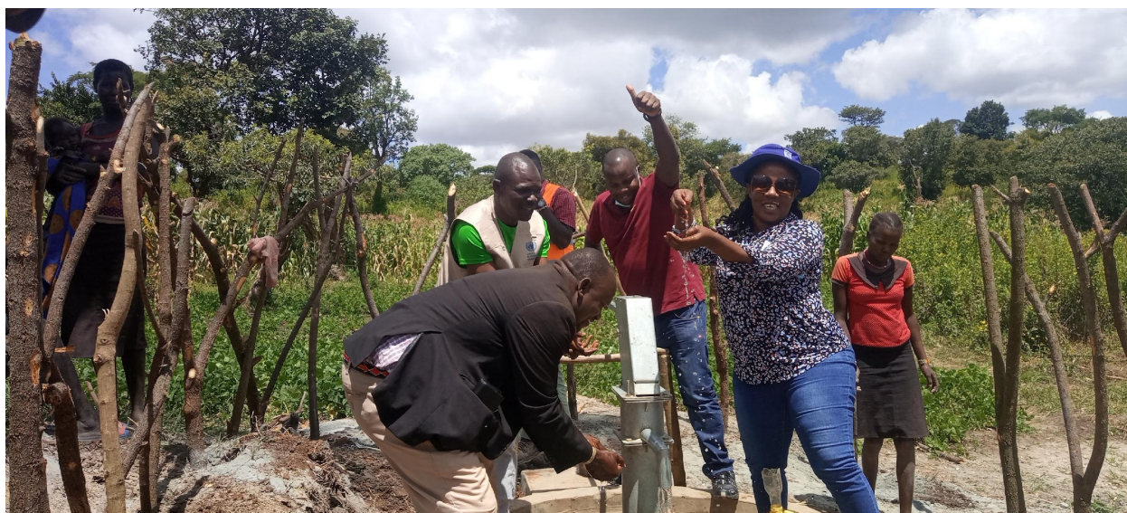
UNDP team and LCV representative – Kaabong testing the newly drilled and installed borehole in Tultul- Timu Sub- County, Kaabong District during the project monitoring - September 2022
