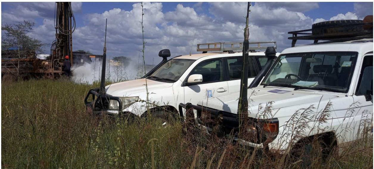
WSF and UNDP vehicles parked during the drilling of a borehole in Kaileny, Nakapelimoru sub-county, Kotido District - August 2022
