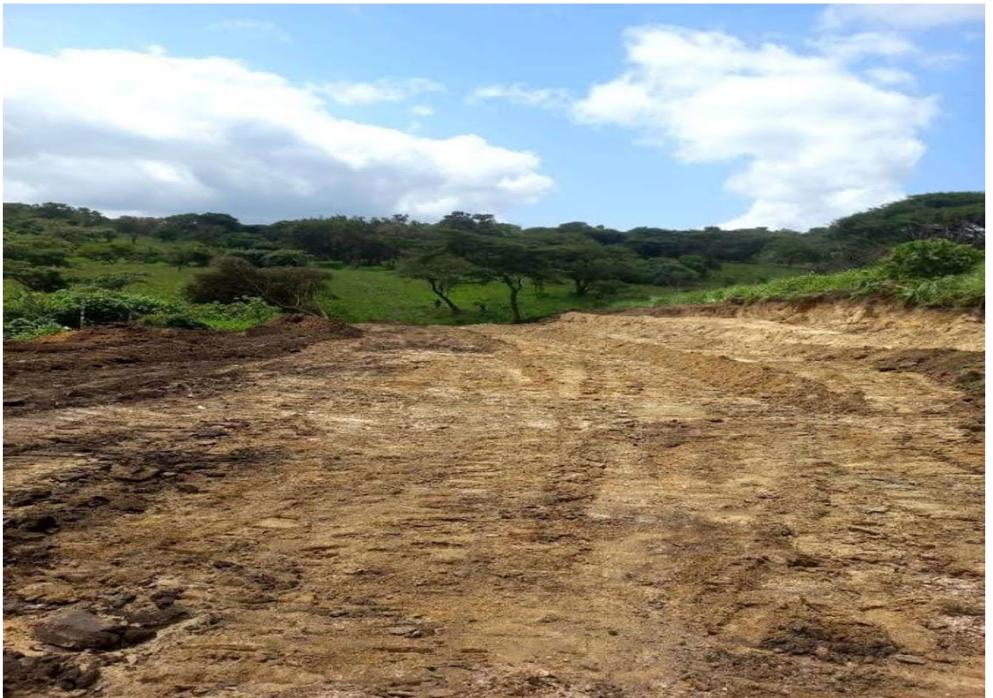
Section of the Loitanit - Kanadap - Nalapatui security access road cleared and opened using a grader.
