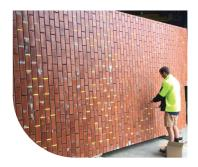
Additionally Form Brick's 'original' form liner system enables every brick wall to have a hand made appearance, with the perp joints randomly imperfect by up to 6mm.
