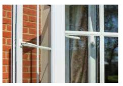
windows. They secure the window at a number of points around the frame, making it more difficult for potential intruders to find a weak point they can exploit to gain entry. Multipoint locks are engaged and disengaged via an espag window handle, which most double glazed windows are fitted with.
