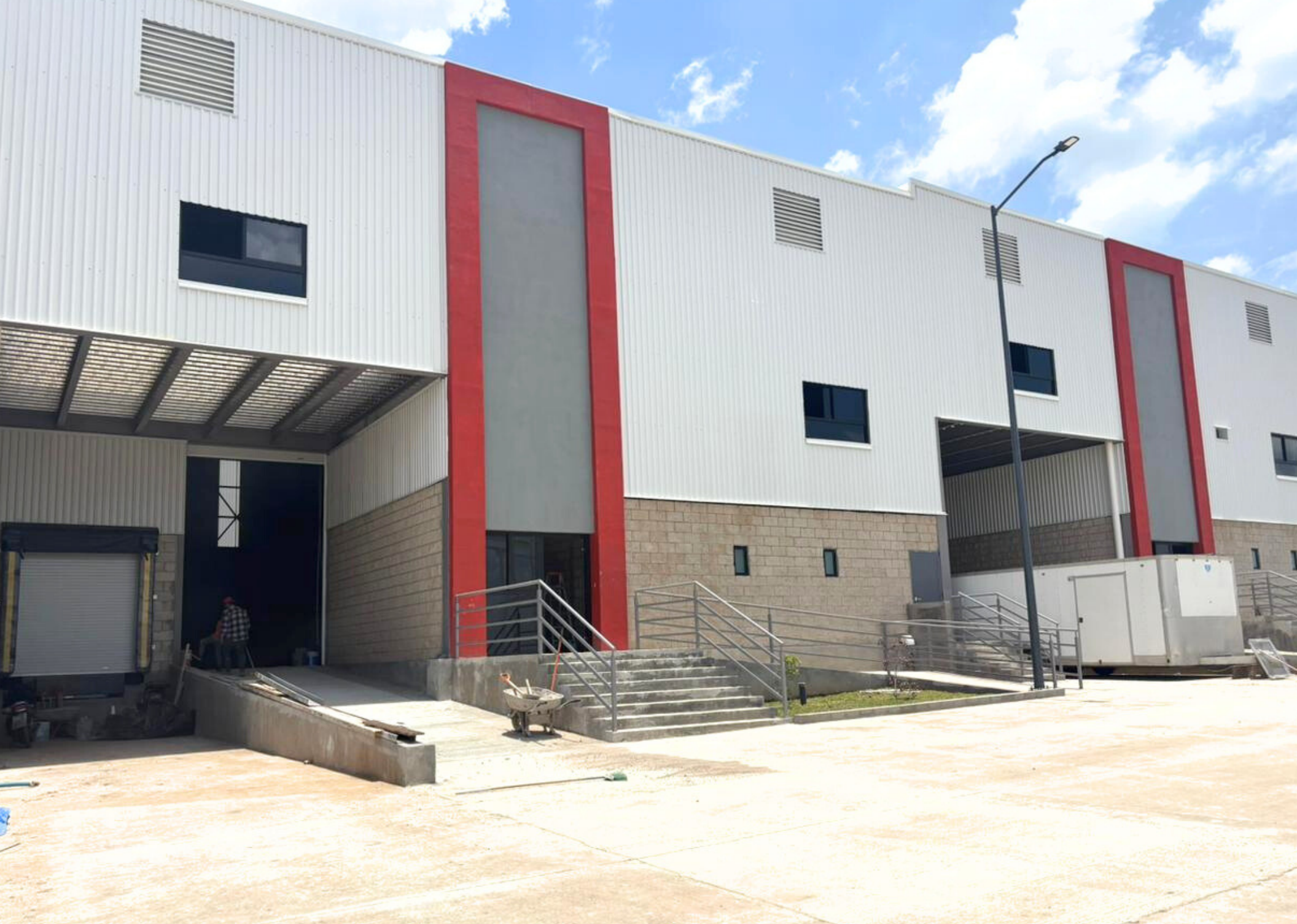
FACHADA NAVE INDUSTRIAL
