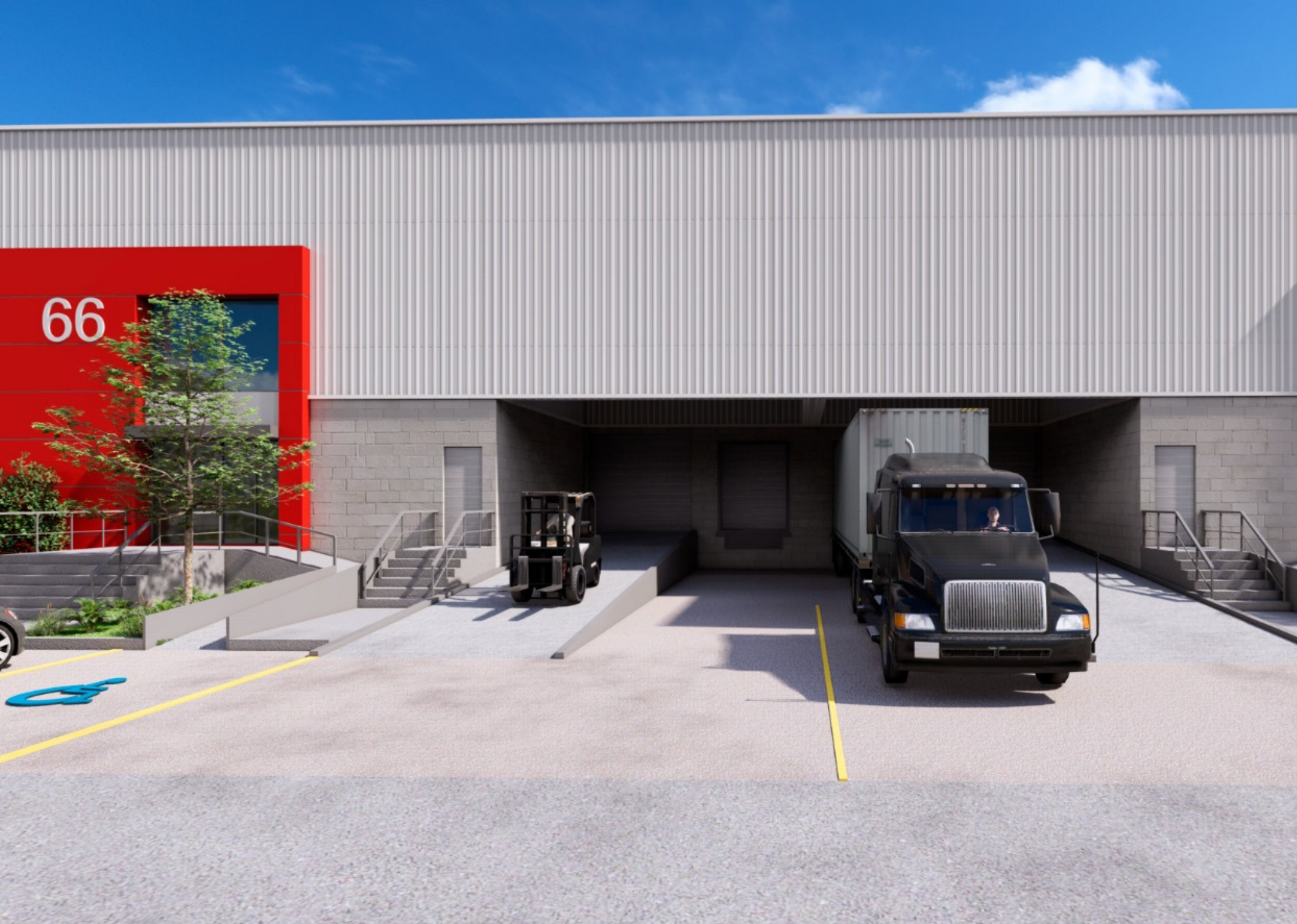
FACHADA NAVE INDUSTRIAL
