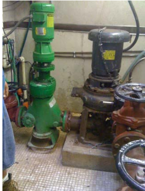
Marina Bay SLS "Before" photo shows High Maintenance Non Clog pump and comminutor. This installation was a constant maintenance headache!
