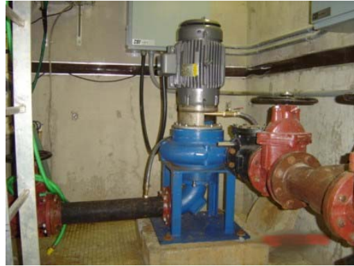
Marina Bay SLS "After" photo shows a dimensionally equivalent ESSCO VDPCC pump installed with comminutor removed which resulted in a very low maintenance and space saving pump station.
