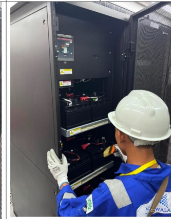
Physical Battery Checking & Cleaning
