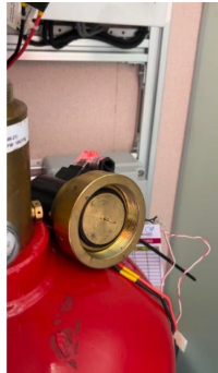
Solenoid Normal Condition
