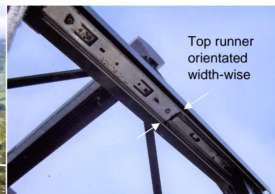
Detail Of The Top Runner 'In-Situ'
