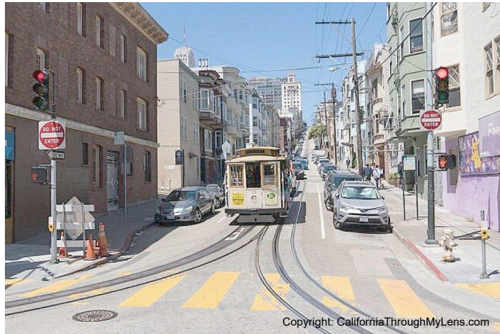
Here is where the line splits, and there will be a cable raising lever in the vicinity. The lines come together and share a centre rail.
