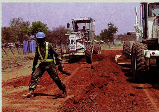
An infrastructure project – ditch-digging
