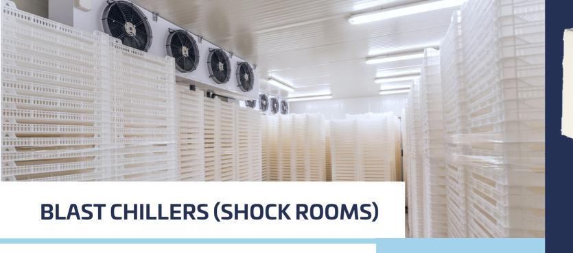
A blast chiller / freezer is a specialised refrigeration unit designed to rapidly reduce the temperature of food products, swiftly bringing them from hot to a safe, chilled state.
