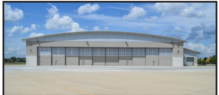
MULTI-PANEL SLIDING HANGAR DOORS
