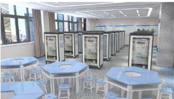
机床电气技能实训室 Machine Tool Electrical Skills Training Room
