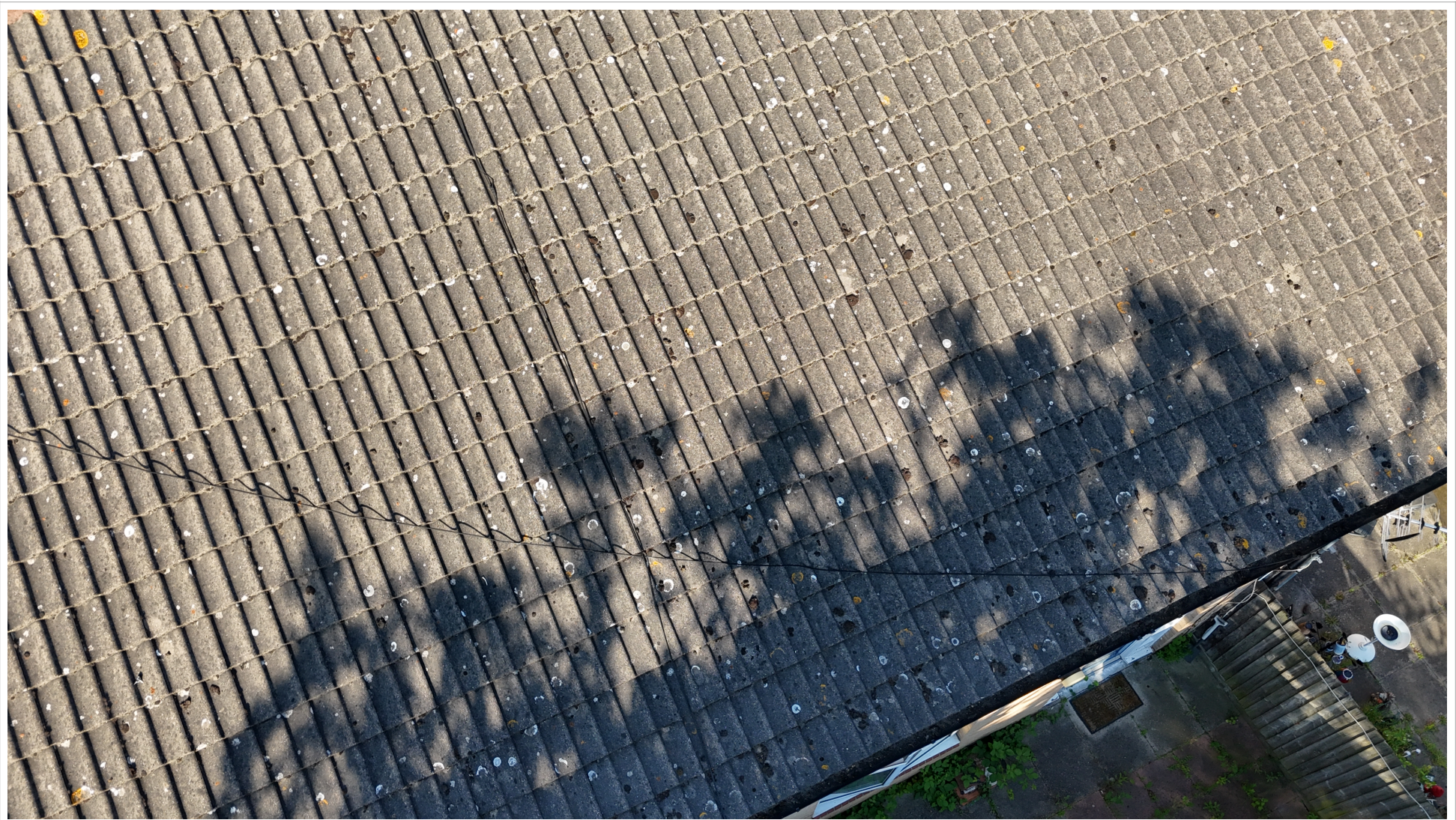
Figure 2: Moss and lichen to rear roof slope
