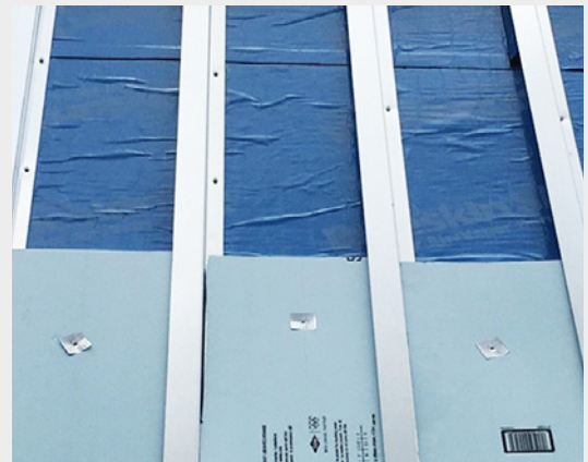
Typical Horizontal Framing
