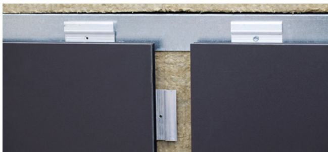
7 Repeat steps 3-5. The next panel is placed onto the J-trim and slid over to connect with the previous panel installed.
