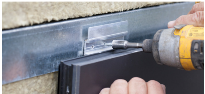
6 The aluminum clip is attached to the sub-framing using a self-drilling hex screw with an extended hex head driver.
