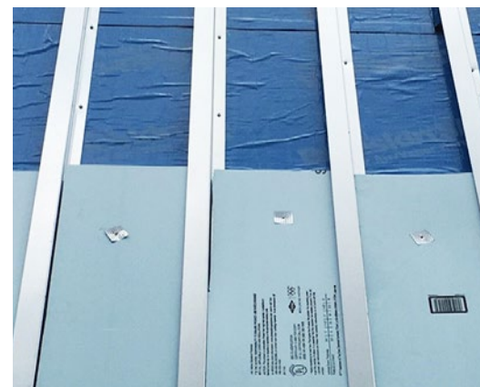
Typical Horizontal Framing
