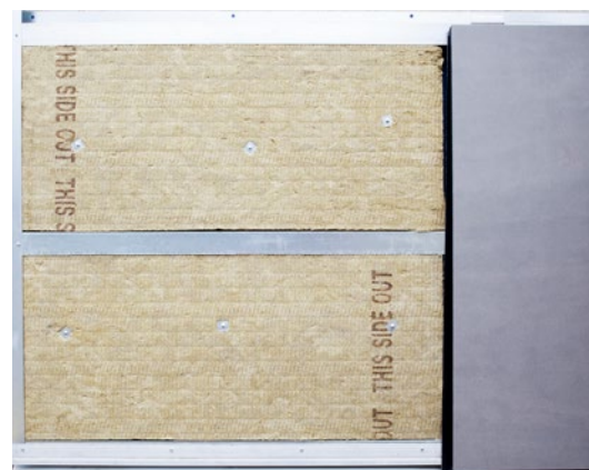
Typical Horizontal Framing
