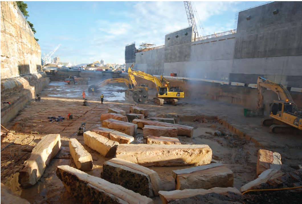
Figure 1-12 Barangaroo Headland Park Foreshore, cutting stone blocks from the onsite extraction hole.
