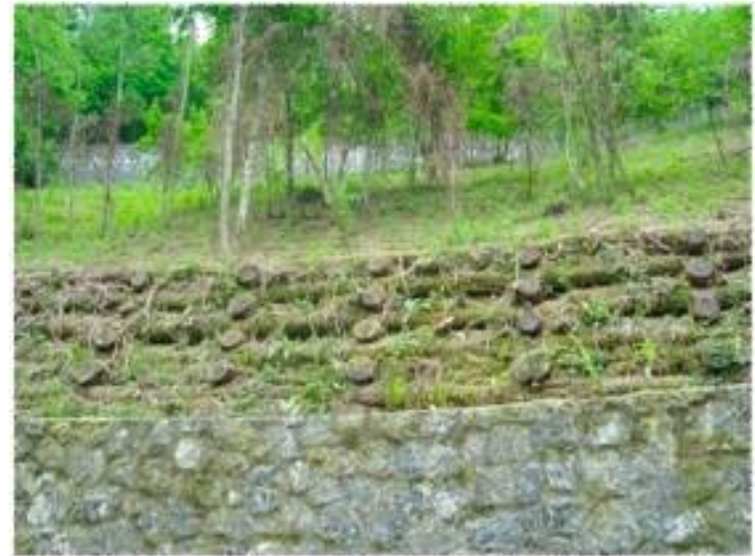
slope crib wall at Desiata, Seravezza (LU), with similar willow cuttings original density
