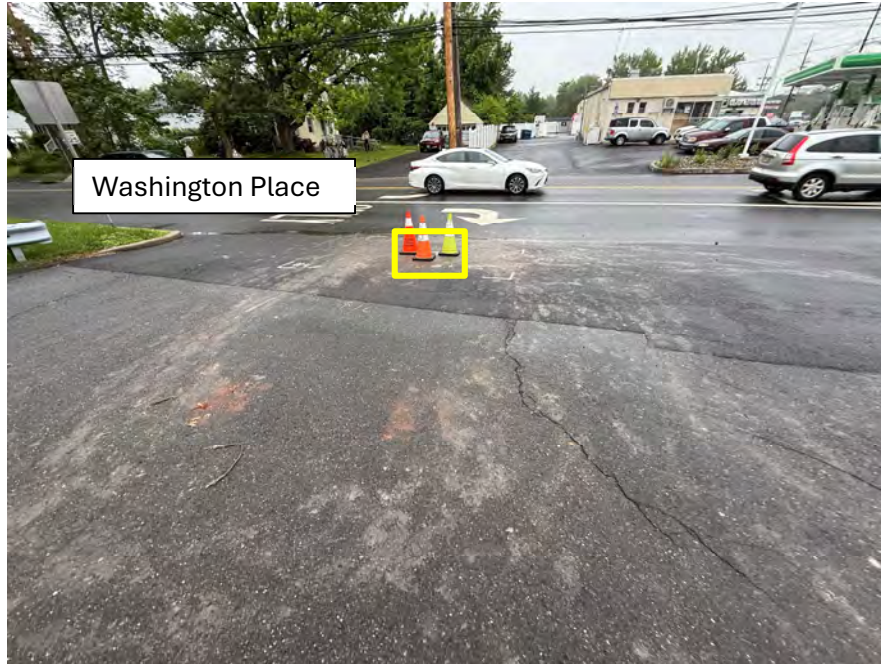
Photograph 11: Picture of MW-3 (MW-3 and 3D) Cluster facing Washington Place from the site property
