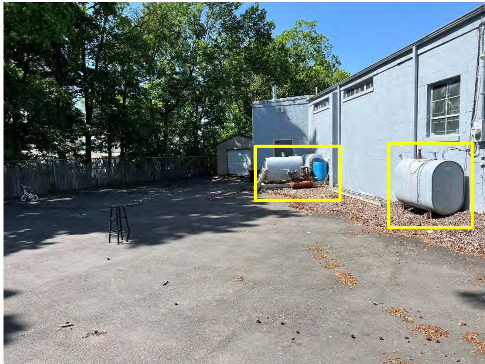
Photograph 2. View of rear parking lot as well as 3 ASTs (Aboveground Storage tanks)
