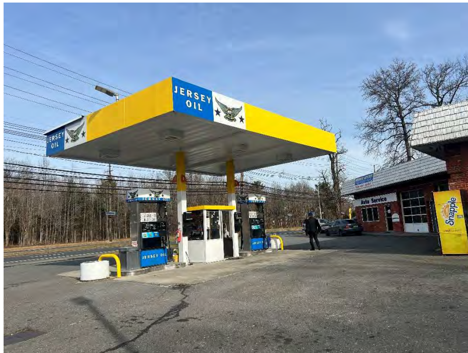
Photograph 10: Fuel pump island facing Route 130.
