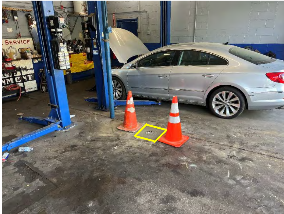
Photograph 3. MW-23 Installed in garage bay area
