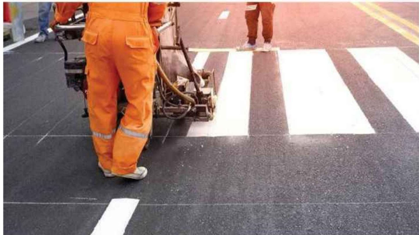
Our range of thermoplastic road markings and signs are permanent, hard surface markings that have been built to last.
