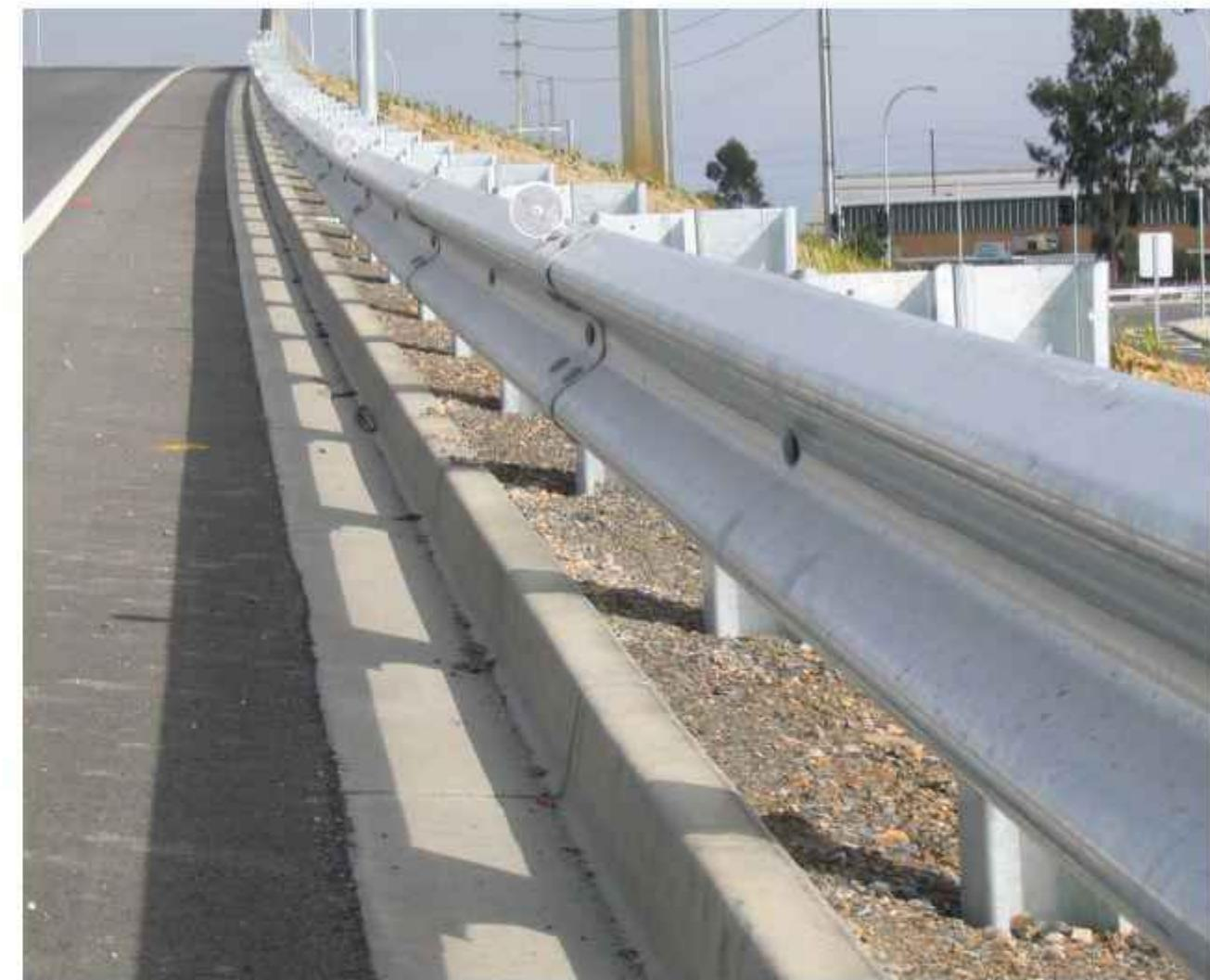
It uses the deformation of the soil foundation, columns, and beams to absorb collision energy and forces the out-of-control vehicle to change direction and return to the normal driving direction to prevent the vehicle from rushing out of the road, protect the vehicle and passengers, and reduce the loss caused by the accident.
