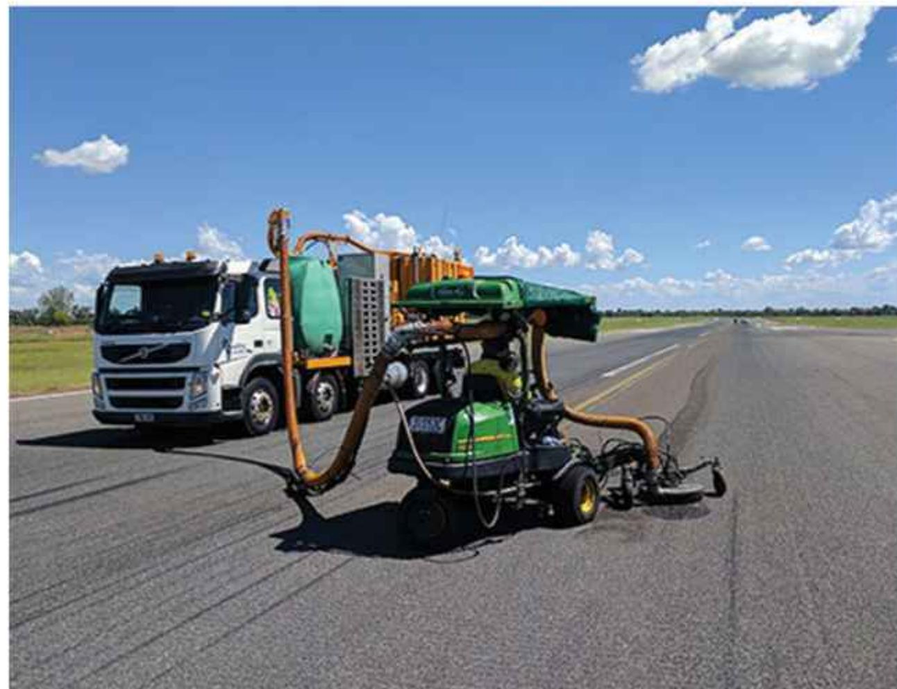
The most common method of removing road markings is grinding. This involves using a specialized machine that grinds the markings down to the surface of the road.
