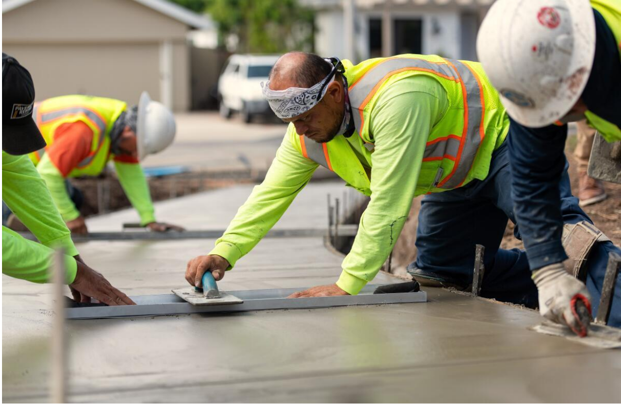
Pedro Gonzalez, center right, and Filemon Muniz, left, press a mold of a poem into a path leading to the playground at Brentwood Park in Costa Mesa. (Eric Licas)
