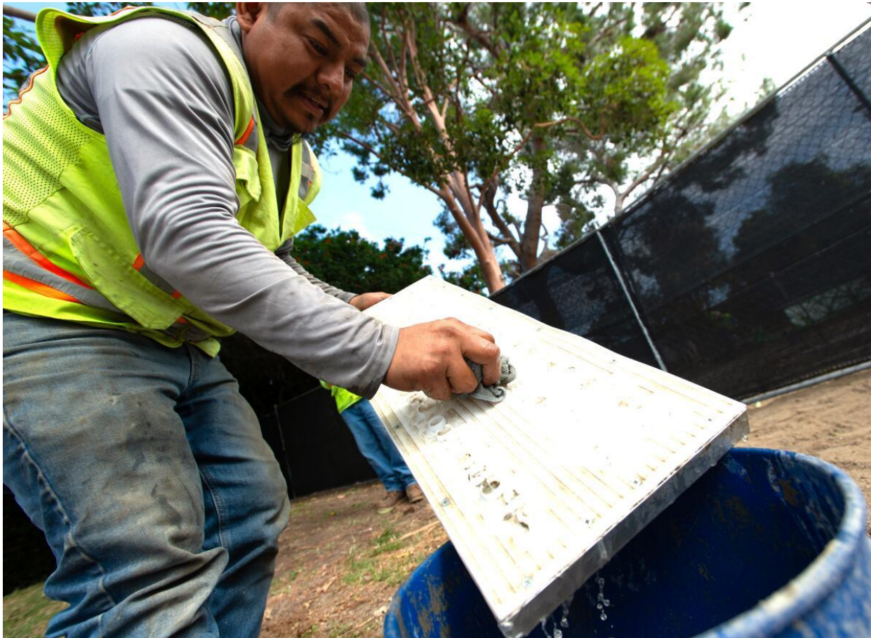
Marco Reyes cleans a mold used to press poems into a concrete path leading to a new playground at Brentwood Park in Costa Mesa. (Eric Licas)
