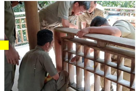
On-Site Restoration & Finishing
