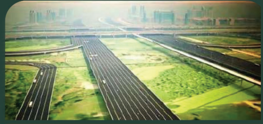
6 Lane Expressway Highway Ahmedabad-Dholera
