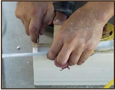
Step 1: Cut the frames as the measured height.
