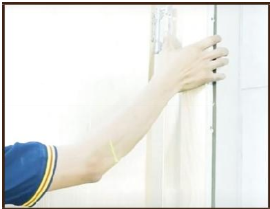
Step 6: Install the door panel to the installed frame.
