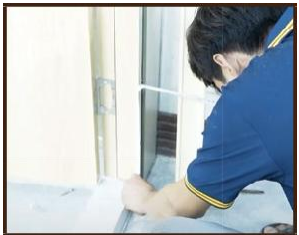
Step 10: Measure and cut the trims, then install them to the frame.
