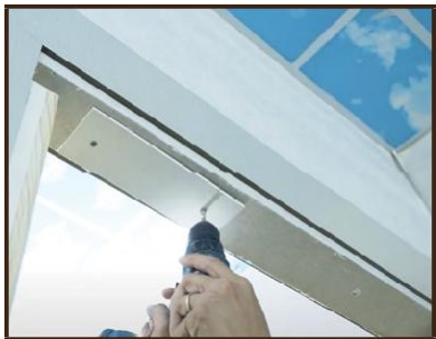
Step 8: Install the horizontal frame.
