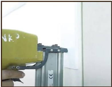
Step 4: Install the hinge side frame first.
