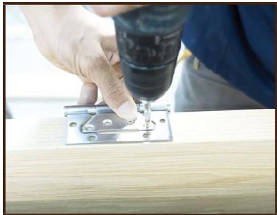
Step 5: Install the 4 hinges to the door panel with the distance shown in the drawing.
