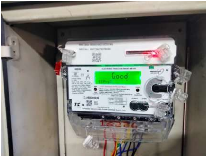
Figure 1: The newly installed Schneider make smart energy meter
