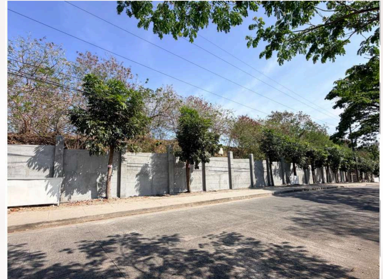
Installation of Perimeter Fence
