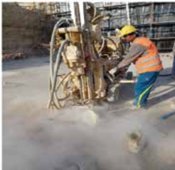
Earthing Drilling Holes- Mallikar Hotel Project Tolkasem Street Riyadh
