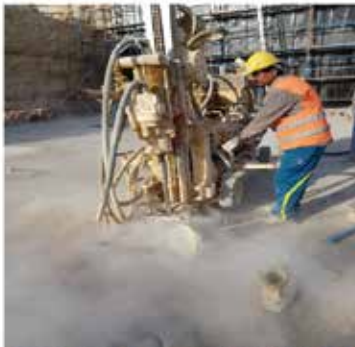
Earthing Drilling Holes- Mallikar Hotel Project Tolkasem Street Riyadh
