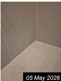
Ref #9.3 - Sealant deteriorated under the basin area
